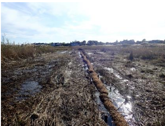
Top Left; Marsh surface prior to drainage channel and runnels, Right Surface after drainage channel and runnels installed, note all the new vegetation growing in previously flooded pannes. Bottom Left; Filling of ditches with coir logs and covered with marsh peat (Right).
